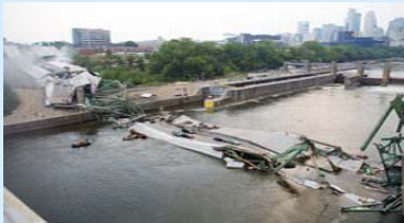
135W Mississippi River Bridge Collapse Minneapolis, Minnesota
