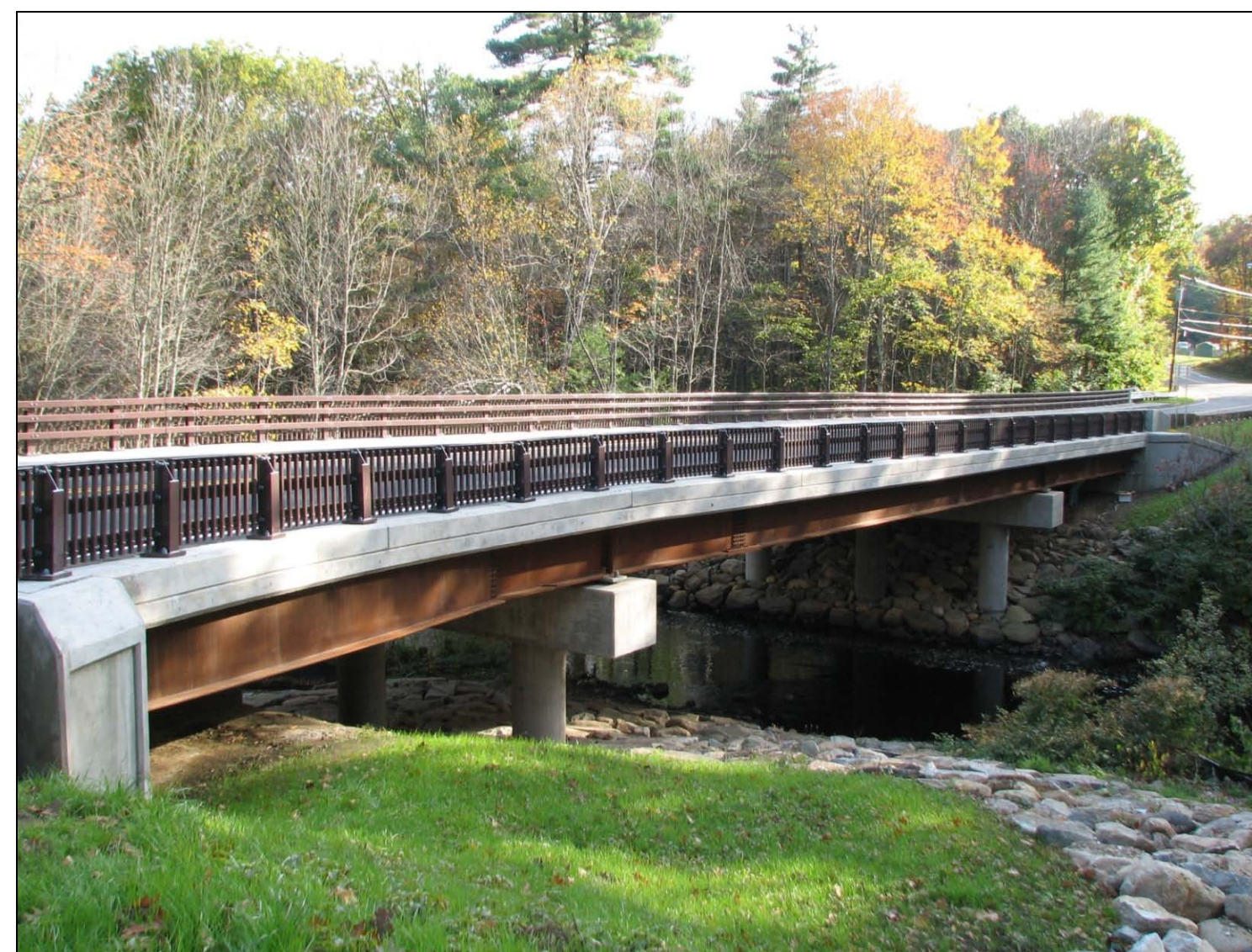
Fig.1 Vernon Avenue Bridge over Ware River – instrumented bridge
