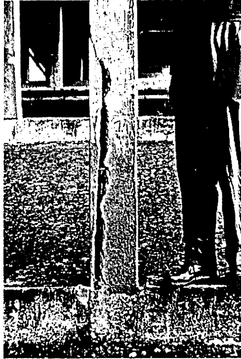
Figure 4: Aarburg Bridge, exposed reinforcement (Baudirektion Aargau, 1967)
